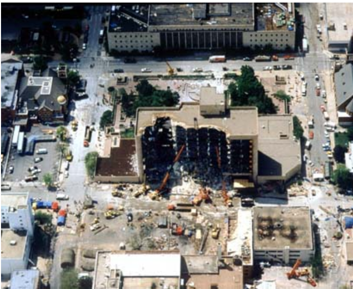
Figure 2-1. Above , Overhead View of Murrah Building Damage 70
