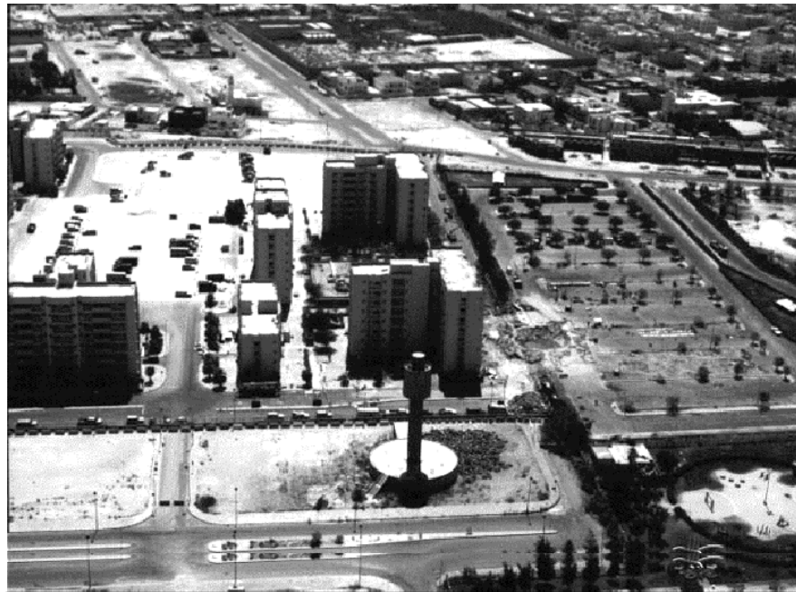
Figure 3-4. Below , Photograph of Khobar Towers After the Bombing (Source: Report to the President and Congress on Protection of U.S. Forces Deployed Abroad (1996).)
